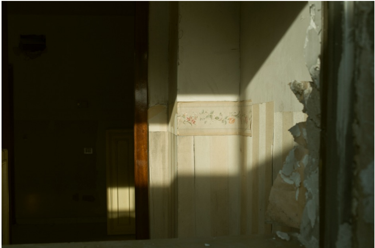
PHOTO 13: details of the wall of a motel room
