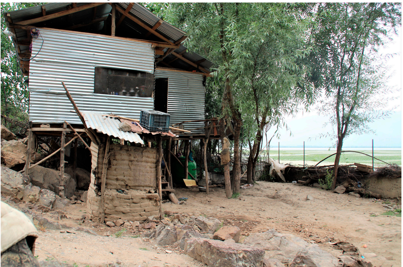
Photo 2 Just a tin shed for the shelter. During the harsh winters, fishermen without the financial means to build a kaccha house build tin shelters on the Government-owned land to keep their families warm. The shed is usually built at a high enough level to avoid being submerged by rapidly rising water.
