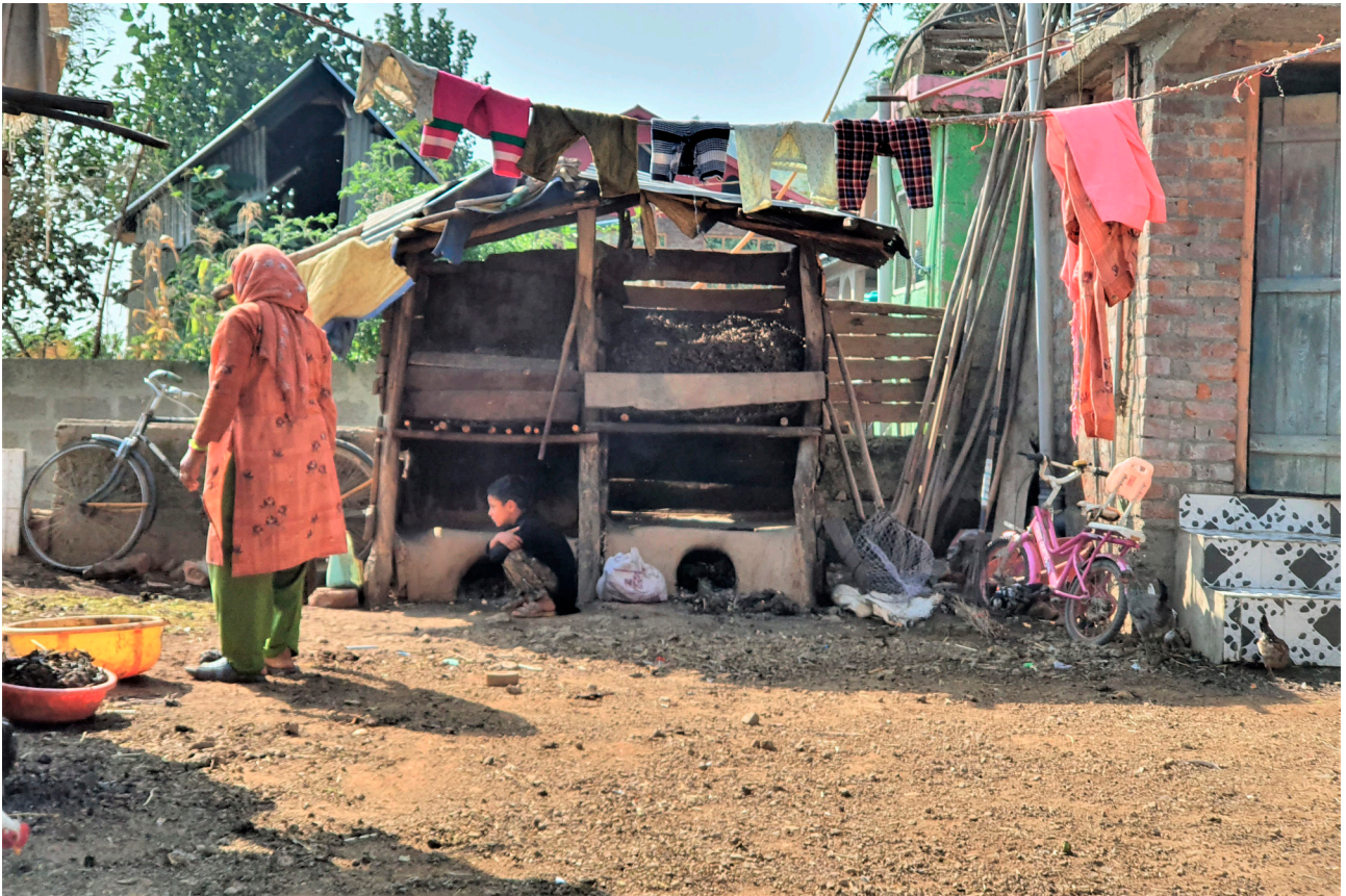
Photo 1 A traditional hearth that serves a dual purpose. Hearths here are mud constructions used for cooking with dung cakes as the fuel source. The upper chamber is intended for storing and drying water chestnuts in harsh winter areas with minimal sunshine, utilising the heat generated by the fireplace. After breaking the dried chestnuts into bits, the top coating is removed. The nuts are crushed into flour and utilised to produce the world-famous Chestnut Tortilla ( gair cxutt ).
