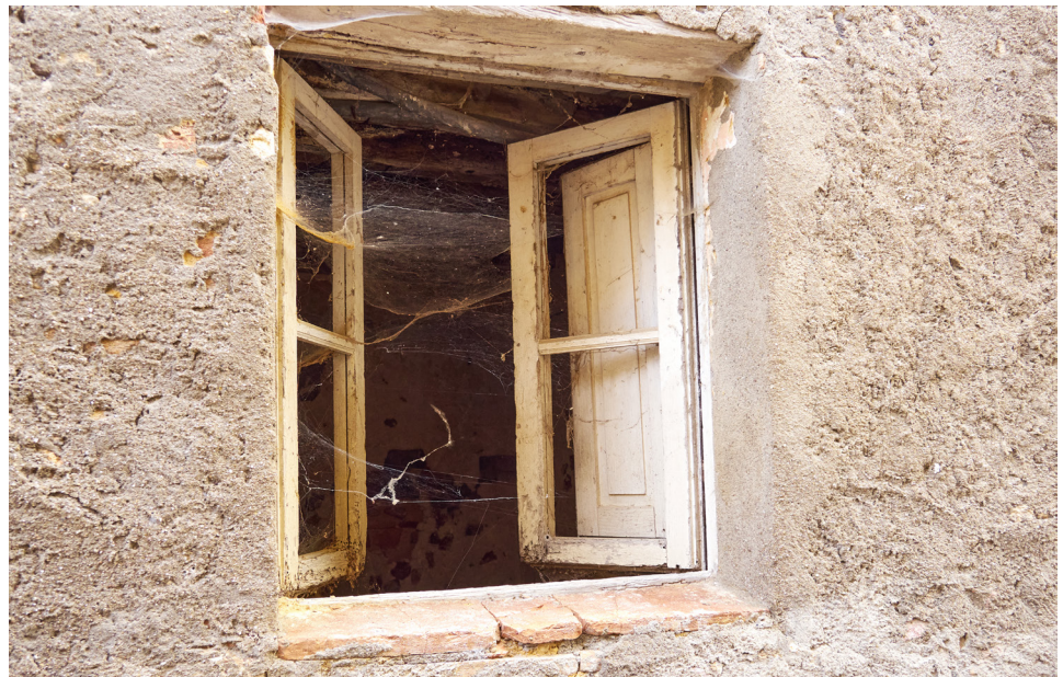
Figure 8 Abandoned house at the centre of Lama (photograph by the authors)
