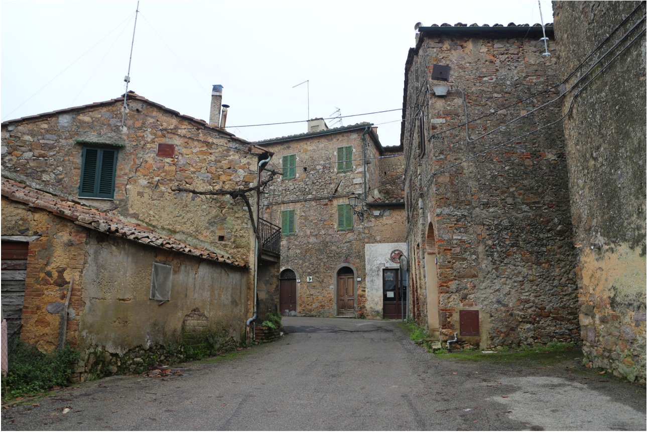
Figure 4 Lama (photograph by the authors)
