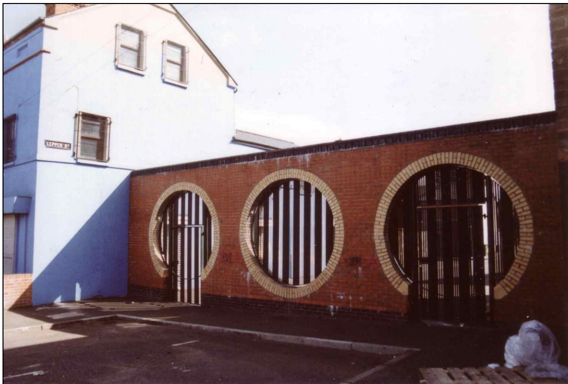
Fig. 14. Security gate, Lepper Street/Duncairn Gardens, view from Duncairn Gardens, after renovation (June 2 nd , 2001) © F. Ballif.
