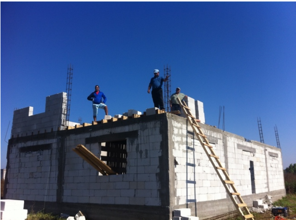
FIGURES 29-30: House under construction
