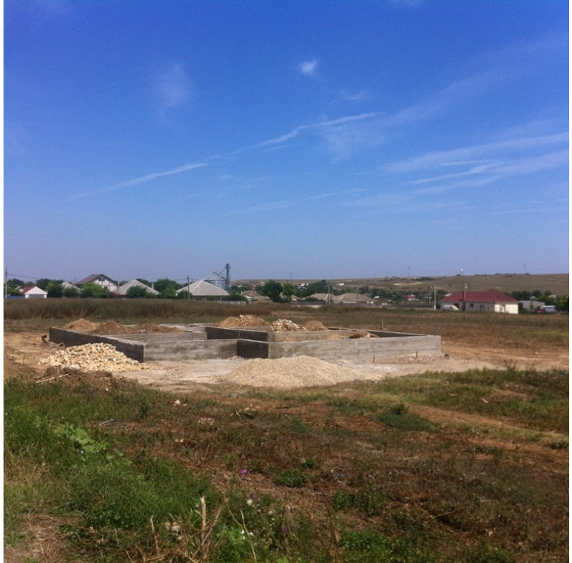
FIGURE 25: Foundations in the new part
