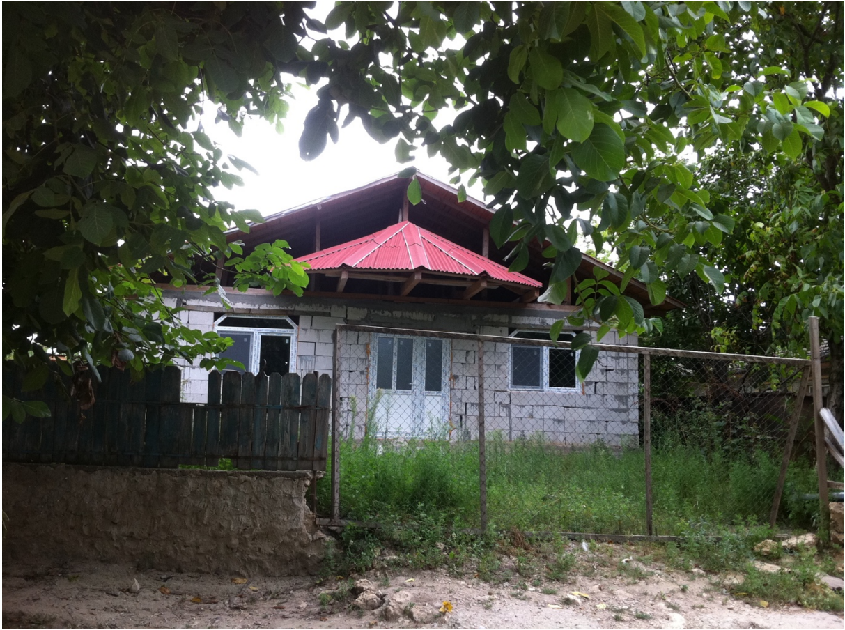
FIGURE 36: House under construction with the first and most important building phase underway
