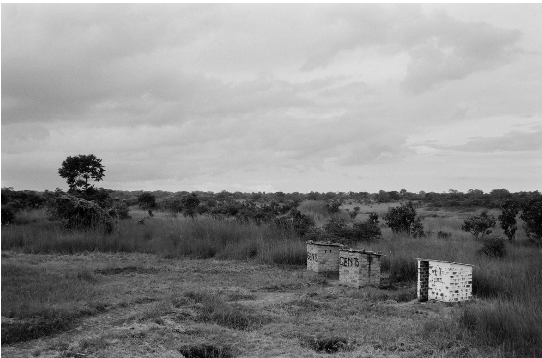
Photo 3: Gents. School restrooms, Block B (2012)
