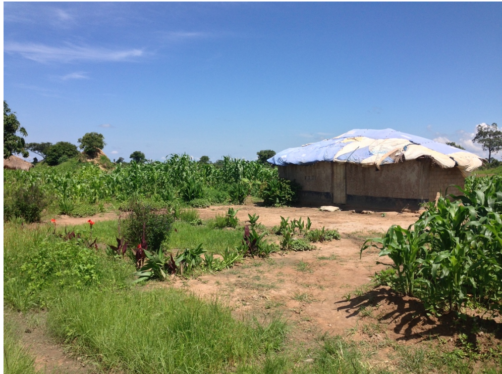
PHOTO 14: UNHCR sheets, House in Block D (2014)
