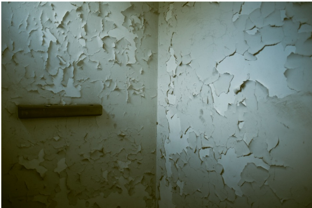
PHOTO 20: Wall of a motel room
