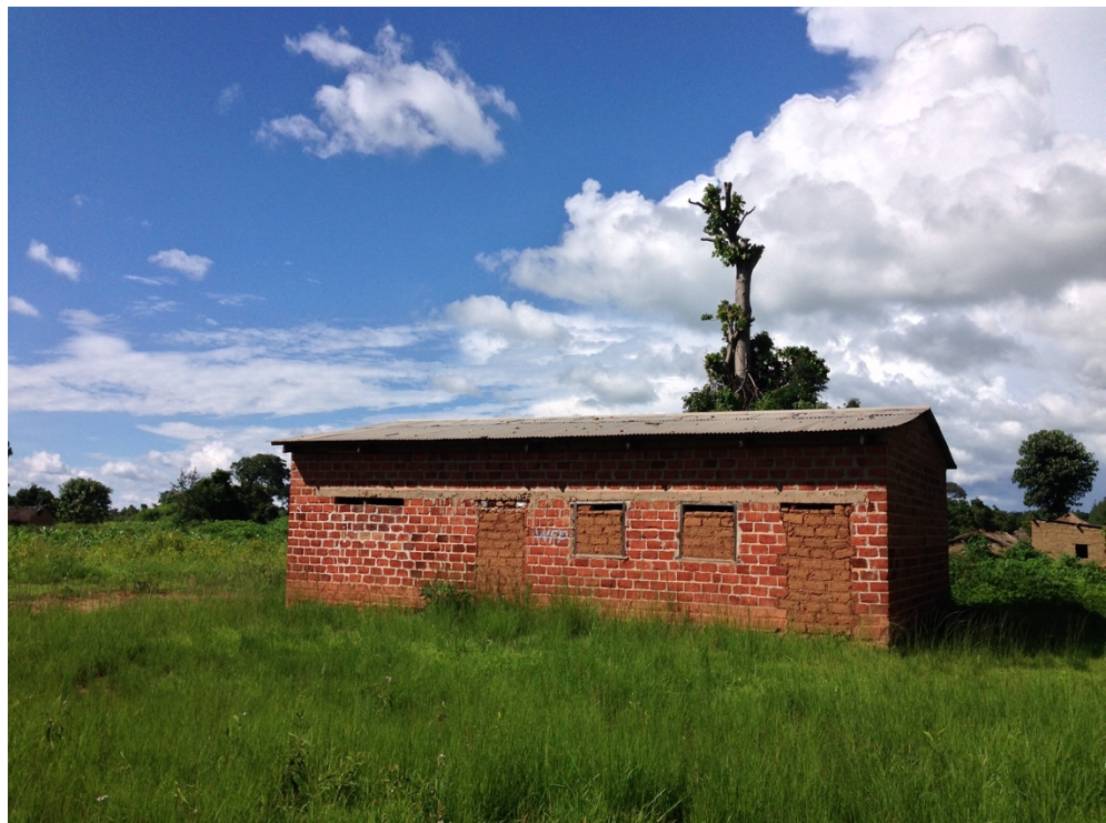
PHOTO 19: Closed doors and windows. Former World Food Program office (2014)
