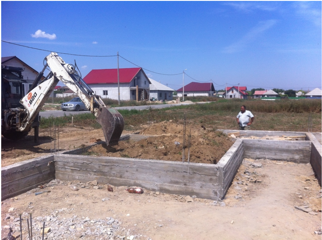
FIGURE 24: Foundations in the new part of the village
