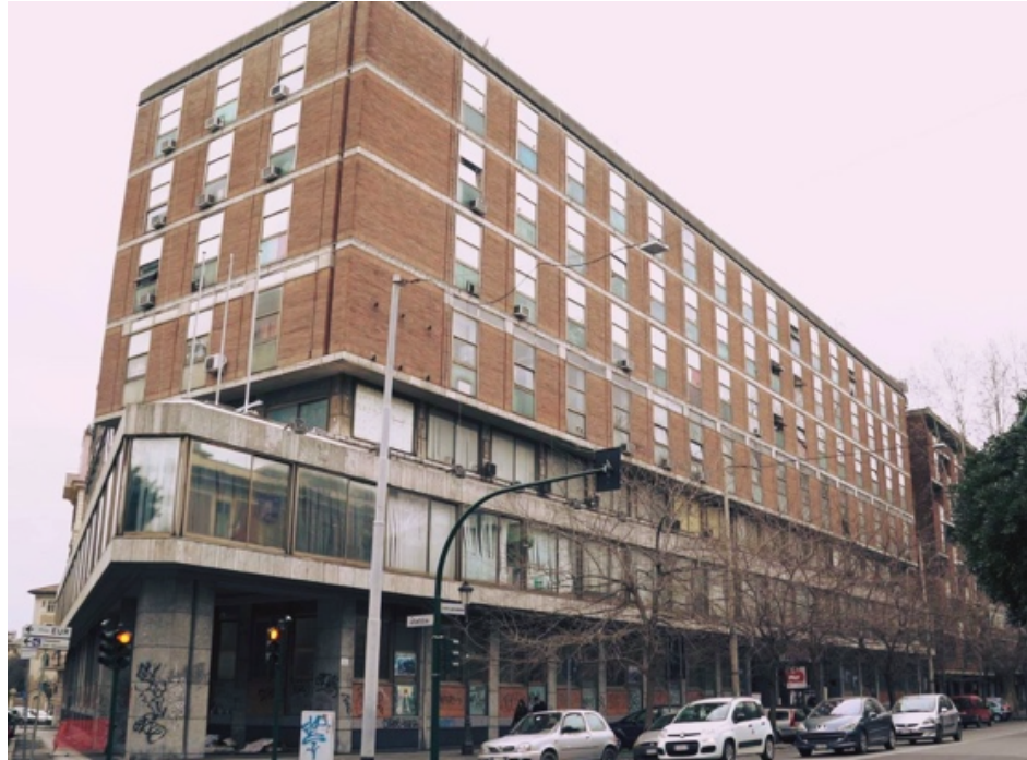
PHOTO 5: The building (Photo by Chiara Cacciotti)
