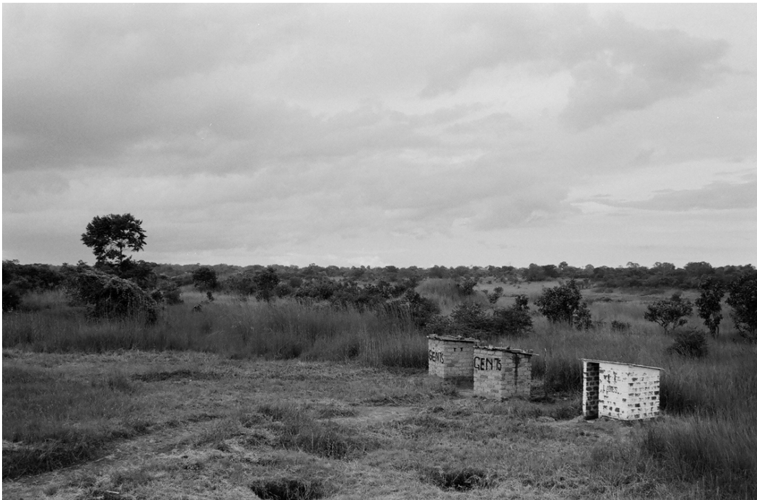
Photo 3: Gents. School restrooms, Block B (2012)
