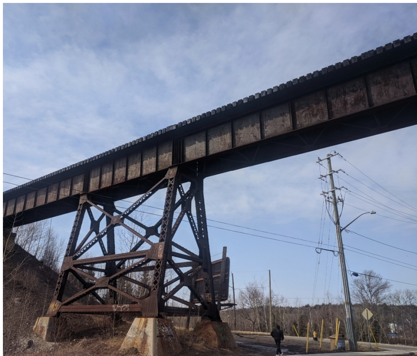
PHOTO 14: The hilly landscape requires bridges for rail. March 2021.
