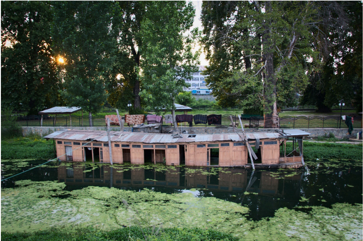
PHOTO 10: Sunked houseboat in Chinarbagh area, Srinagar. Houseboats, once filled by tourists coming from over the world, nowadays are often empty due to the turmoil. In Kashmir the tourist business in general has been deeply affected since the armed struggle has started in 1989.
