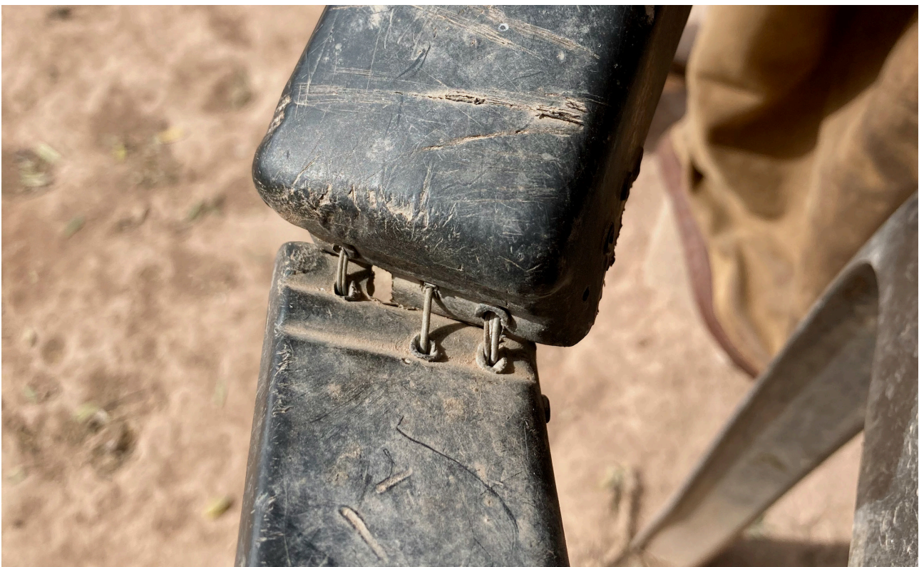
Photo 1 The broken armrest has been sewn together with iron wire. The fact that the chair is less comfortable and that the armrest does not serve to support the arm is secondary to the fact that the chair remains intact. The armrest has therefore lost its primary function, but this does not prevent the chair from continuing to serve.
