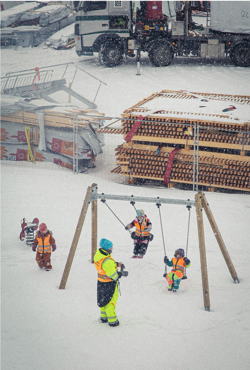
Figure 19 Children playing next to a construction site (Svalbard). Photo by Tomas Salem, May 2021
