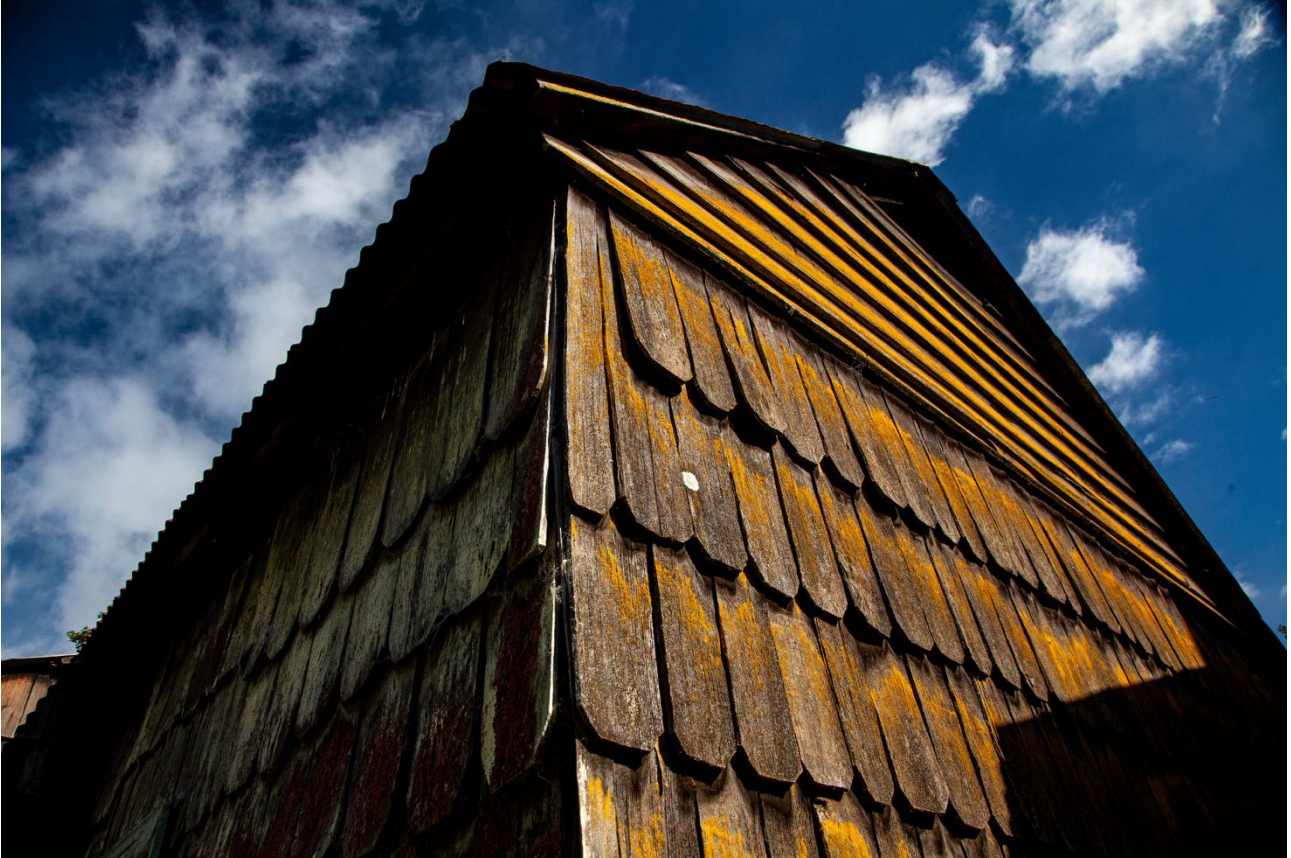
Figure 9 Alerce shingles with yellow and red lichens in Cochamó. Photo by Pablo Fernández, 2022.
