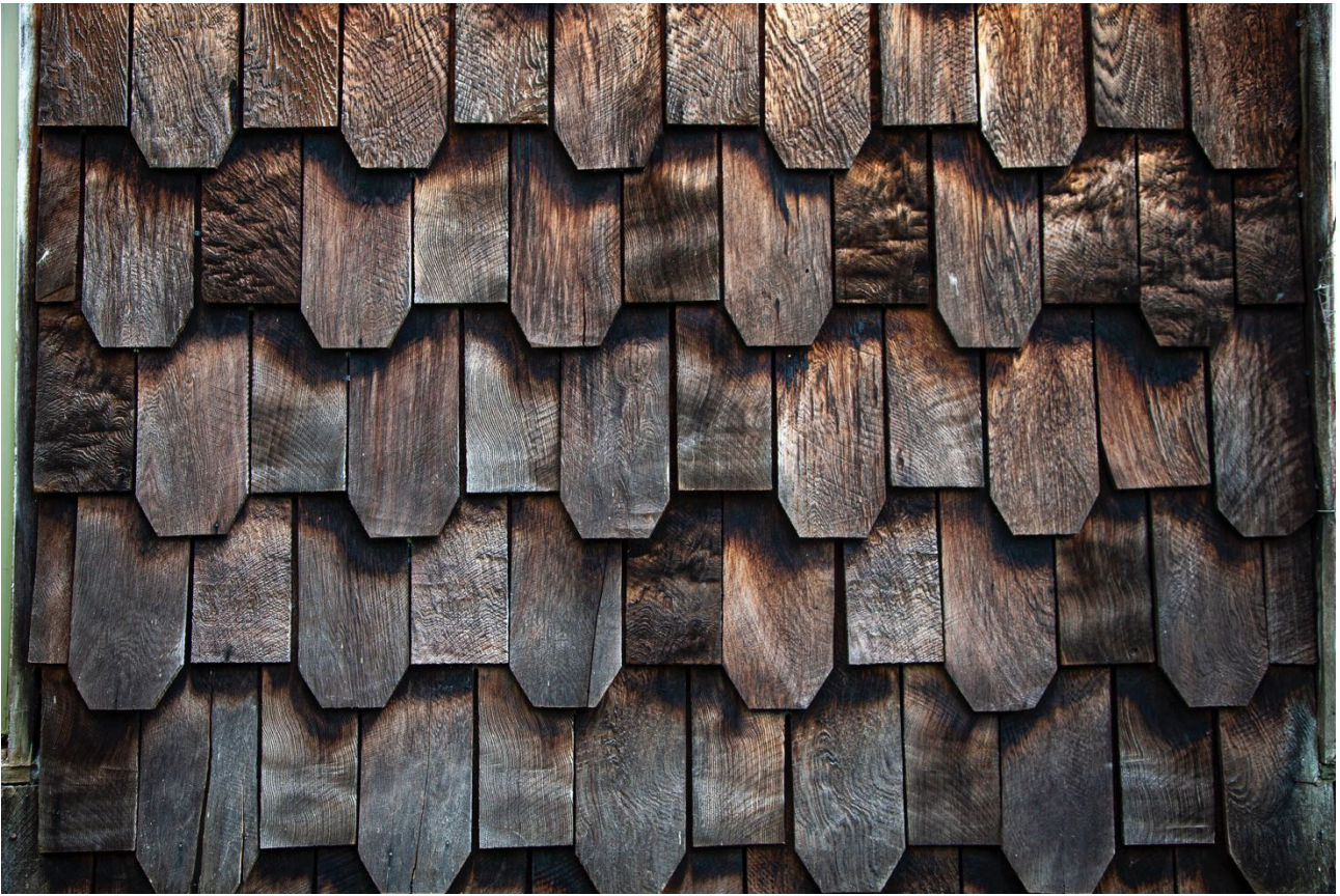
Figure 5 Alerce shingles on the Binational House, Paso El León. Photo by Pablo Fernández, 2023.
